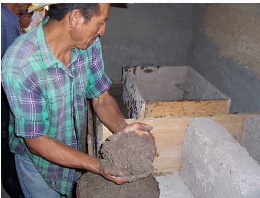
Placing mud in form
