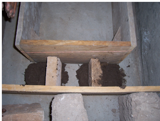
Placing bricks in place for air-wood entry
