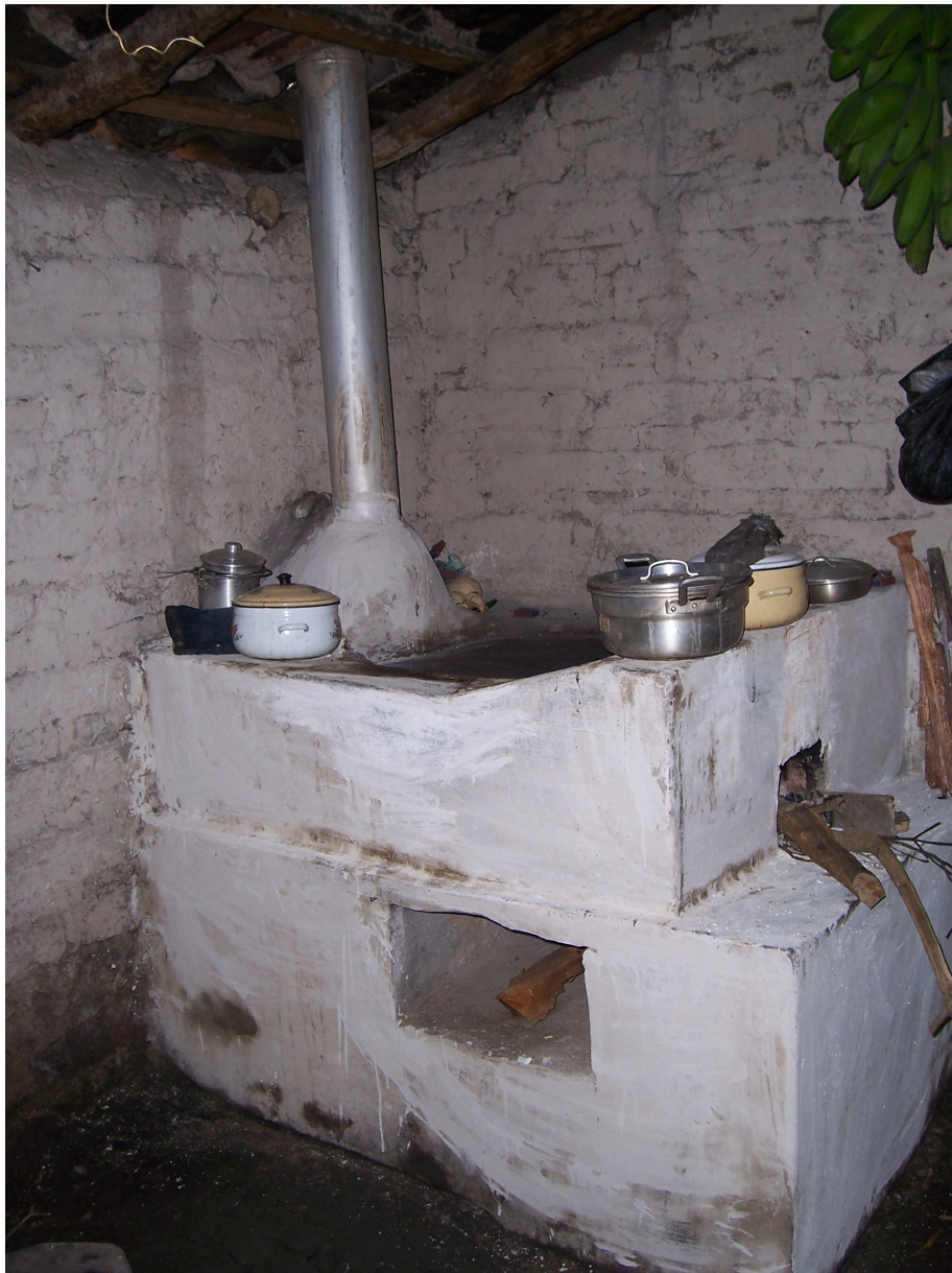
Improved cook stove in operation six months after construction
