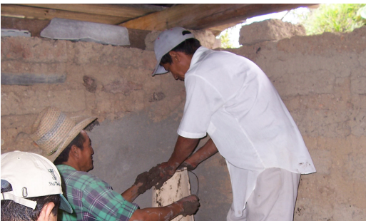
Placing mud in form
