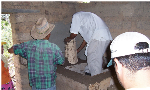
Placing barb wire in form
