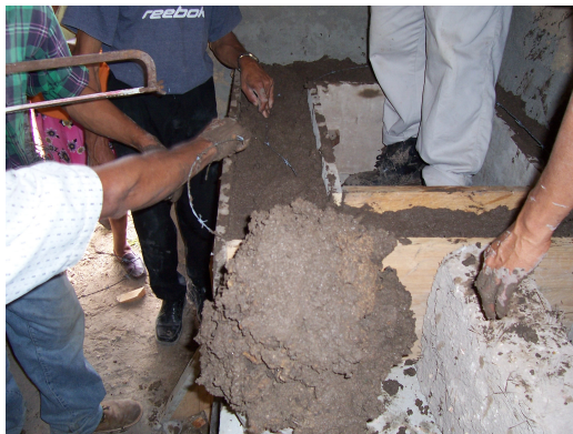
Placing barb wire in form
