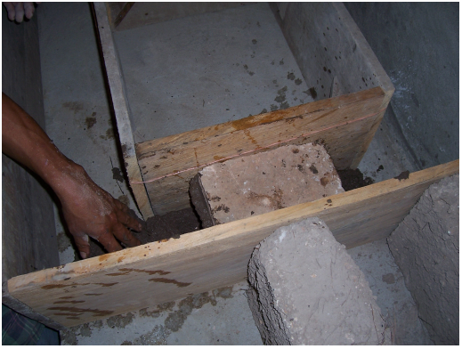
Placing mud around bricks to seal in place
