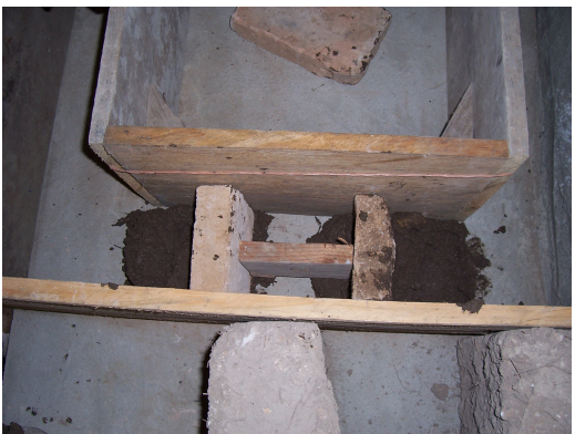
Wood spacer holding bricks in place
