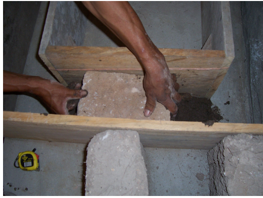
Placing top brick in place
