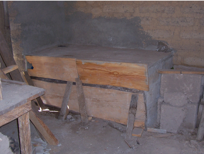
Mesa built of cement drying
